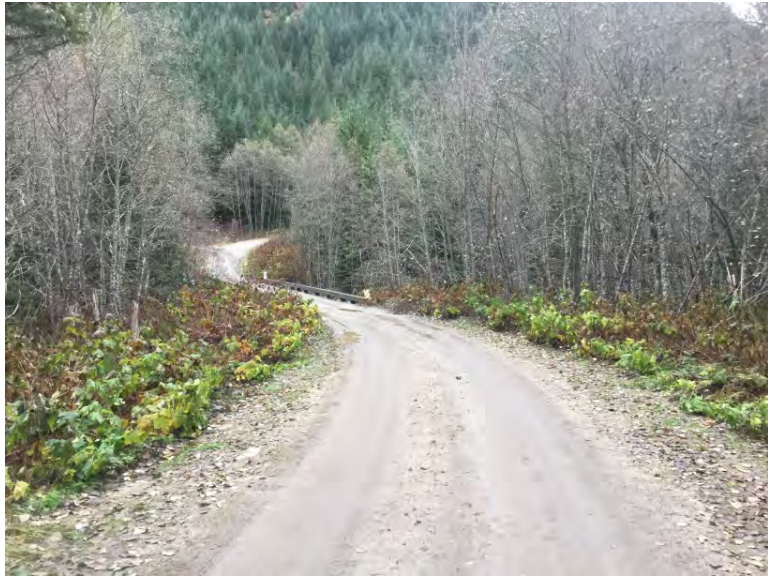
Approach from Left Bank when facing downstream
