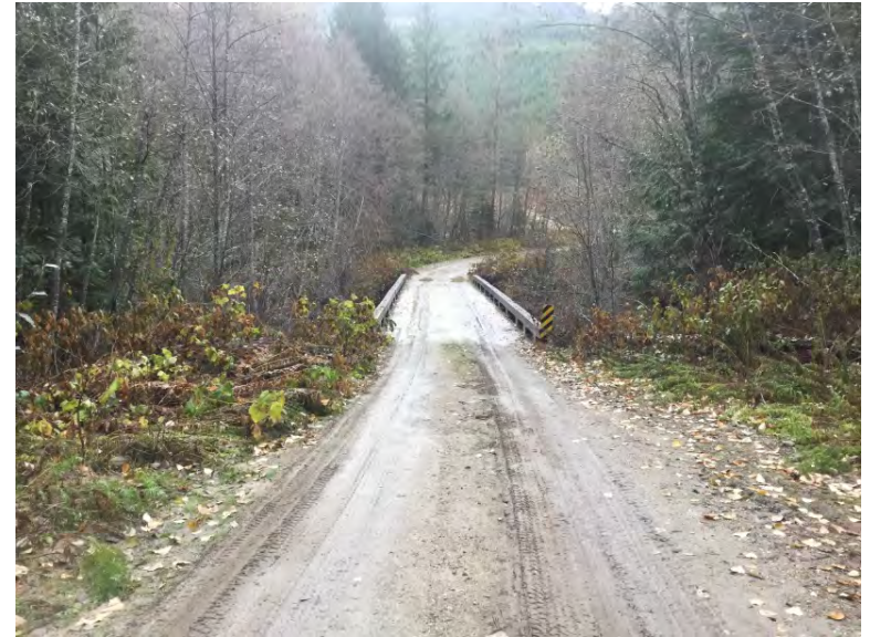
Approach from Right Bank when facing downstream
