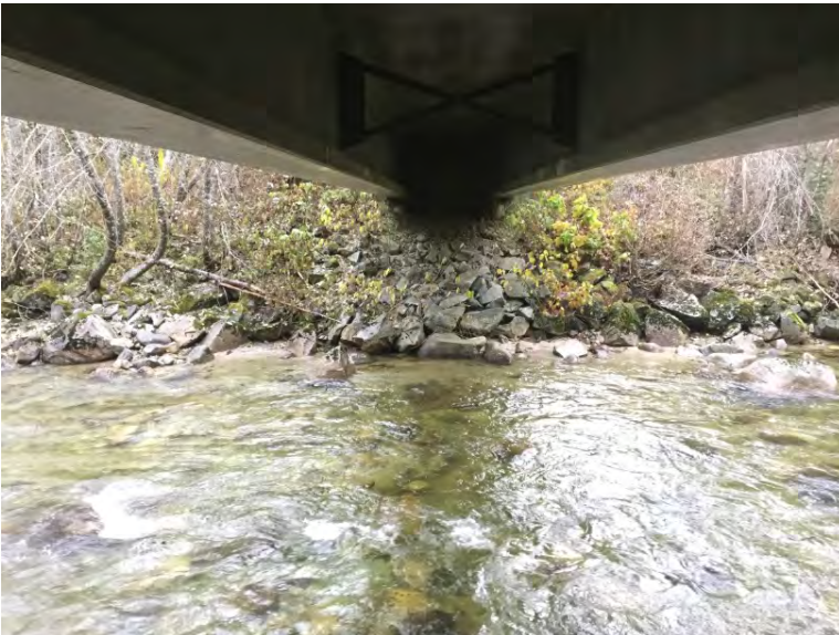
Left Bank Abutment when facing downstream
