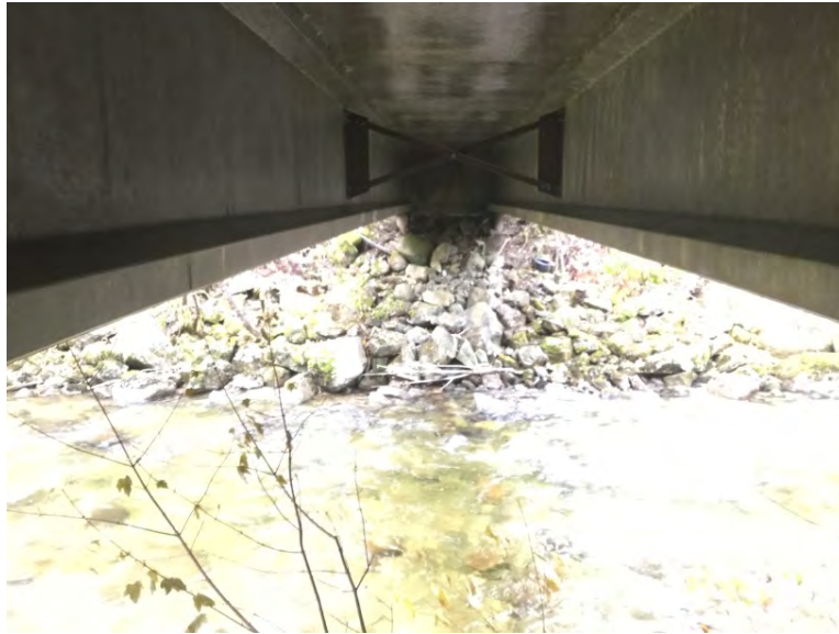
Right Bank Abutment when facing downstream
